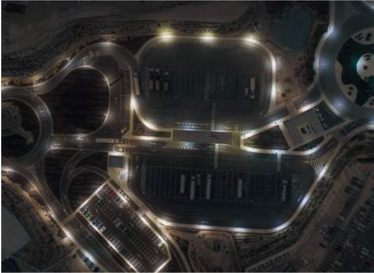
→ LED lighting throughout the Cosentino industrial park
